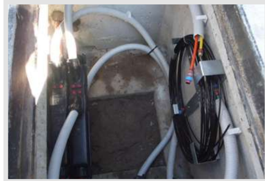
Placing microcables on a cable reserve frame
