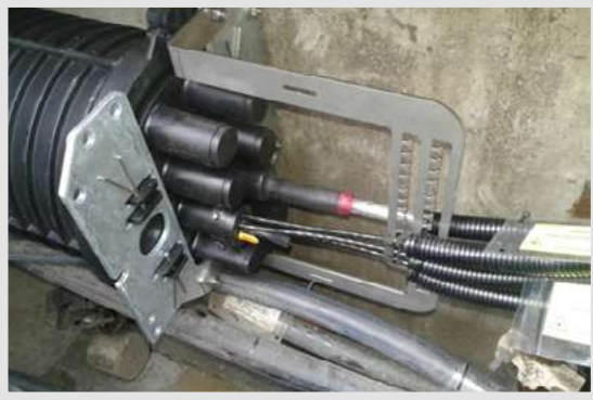
An example of placing a microduct system to a cabinet
