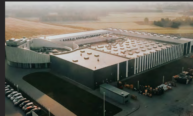
FIBER OPTIC TECHNOLOGIES & PHOTONICS MANUFACTURING LABORATORY CENTER IN ZACZERNIE (I)
